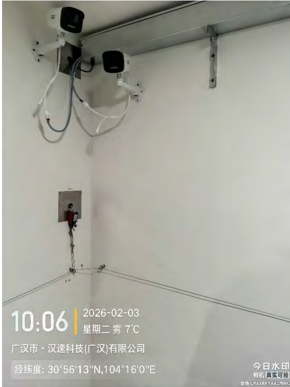
(a) 辐照室拉线开关
